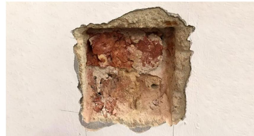
(Above) Plaster sampling at one of the columns in St Andrew's Cathedral. A sample of the plaster was taken from the surface to the brick substrate for laboratory analysis. In this photograph, a thin layer (2–3 mm) of grey Portland cement screed can be seen under the white paint layer. Courtesy of Yeo Kang Shua.
