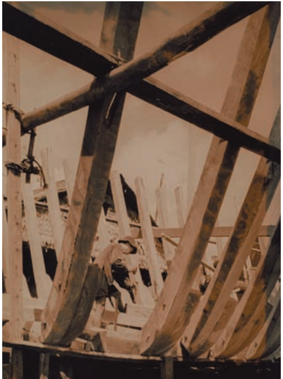
Constructing a tongkang
