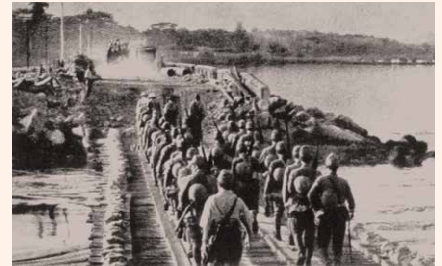
On 31 January 1942, British troops set off two explosions on the Causeway. The first wrecked the lock’s lift-bridge, while the second caused a 70-foot gap in the structure. This photo shows Japanese troops crossing the Causeway into Singapore after constructing a girder bridge over the gap. Lim Kheng Chye Collection, courtesy of National Archives of Singapore.
