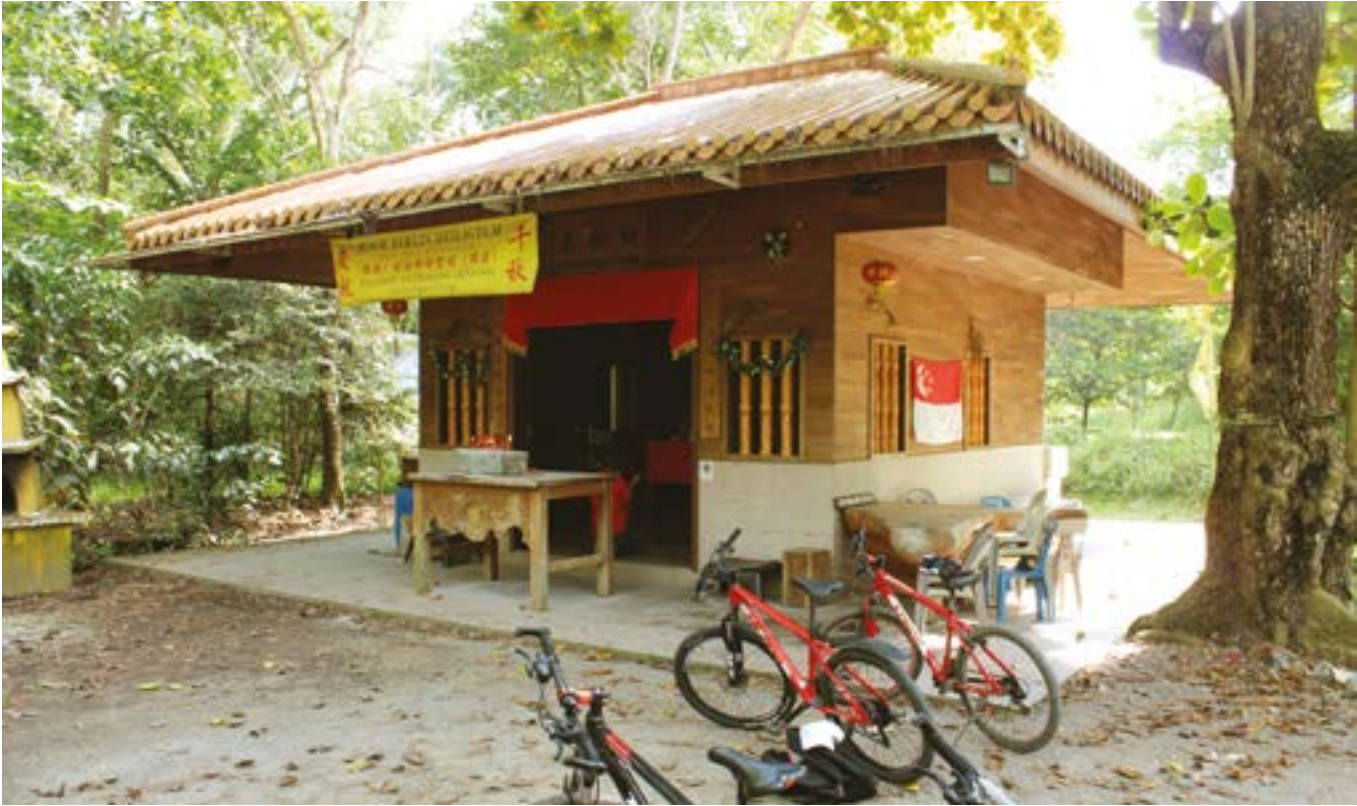
After an extensive renovation in 2015, the 12-square-metre German girl shrine on Pulau Ubin is today a slightly larger brick structure with granite cladding, a tiled roof and ceramic bamboo window bars, 2021. Courtesy of William L. Gibson.
