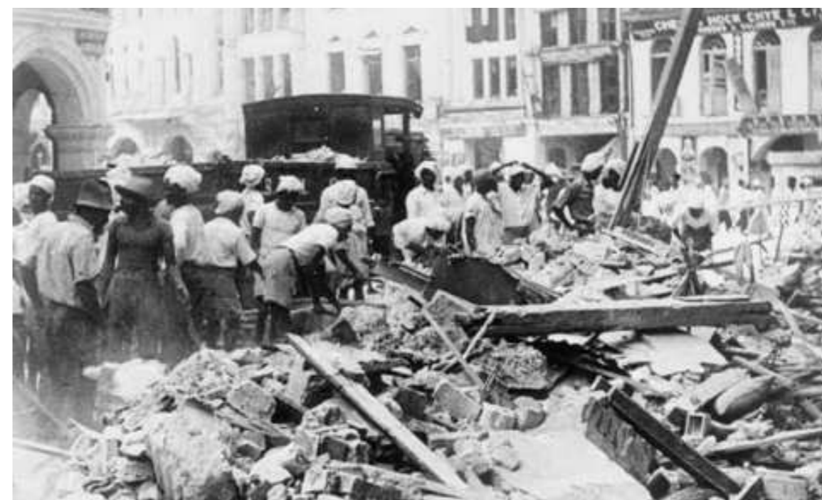
Indian labourers clearing debris in Singapore after a Japanese air raid, 1942. © IWM (HU 57224).
