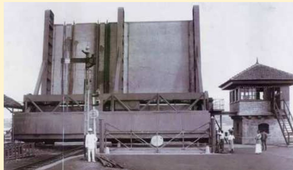
The lock channel at the Johor Bahru end of the Causeway showing the rolling lift-bridge in open position, level-crossing gates and the operating cabin, June 1924. The lift-bridge was electrically operated by a 35-horsepower motor but could also be manually operated. The level-crossing gates placed on both sides of the lock were mechanically operated and were controlled from the operating cabin. The speed limit in 1924 was 10 mph. Courtesy of National Archives of Malaysia.
