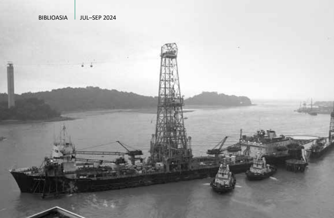
The Eniwetok after its collision with the cableway, 1983. Source: The Straits Times © SPH Media Limited. Reprinted with permission.
