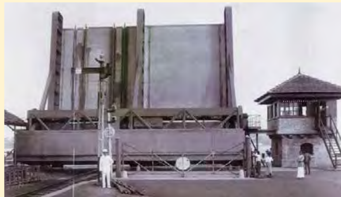
The lock channel at the Johor Bahru end of the Causeway showing the rolling lift-bridge in open position, level-crossing gates and the operating cabin, June 1924. The lift-bridge was electrically operated by a 35-horsepower motor but could also be manually operated. The level-crossing gates placed on both sides of the lock were mechanically operated and were controlled from the operating cabin. The speed limit in 1924 was 10 mph. Courtesy of National Archives of Malaysia.
