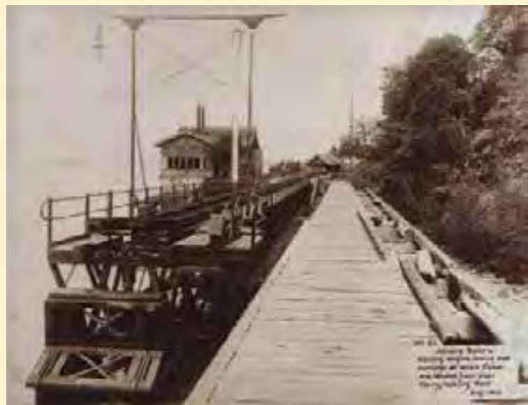
The wagon-ferry jetty in Johor Bahru, August 1919. The hauling engine house or powerhouse on the left contained the winding machinery for hauling travellers to and from the wagon-ferries. Courtesy of National Archives of Malaysia.
