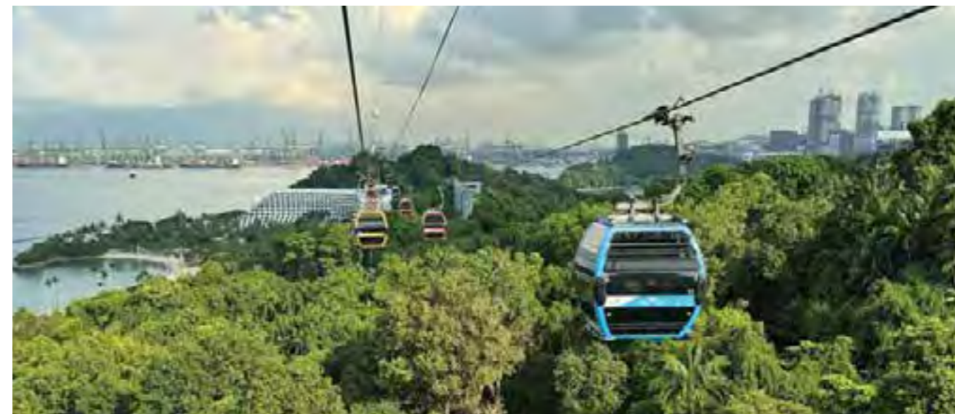
Completed in 2015, the Sentosa Line serves passengers within Sentosa with three stations: Merlion Plaza, Imbiah Lookout and Siloso Point. Photo by Jimmy Yap.
