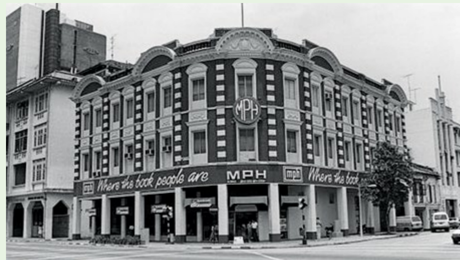
The Edwardian-style Methodist Publishing House building at the junction of Stamford Road and Armenian Street opened in 1904. It was subsequently renamed Malaya Publishing House and then Malaysia Publishing House. MPH bookshop has since moved out of this location, but for nearly a century this was the grand dame of the bookshop scene in Singapore. (The Singapore Management University currently leases the building.) This 1984 image is from the Lee Kip Lin Collection. All rights reserved. Lee Kip Lin and National Library Board, Singapore 2009.
