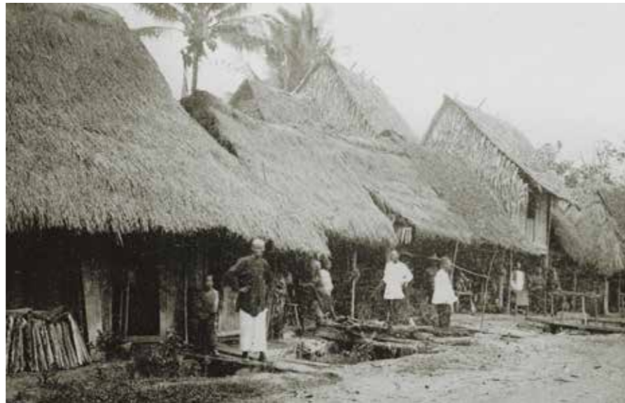
A 1915 photo by G. R. Lambert & Co. showing some attap houses in a kampong, possibly at Bukit Timah. Mangrove habitats also host nipah palms, whose leaves are used for thatching. Lee Kip Lin Collection. All rights reserved. Lee Kip Lin and National Library Board, Singapore 2009.
