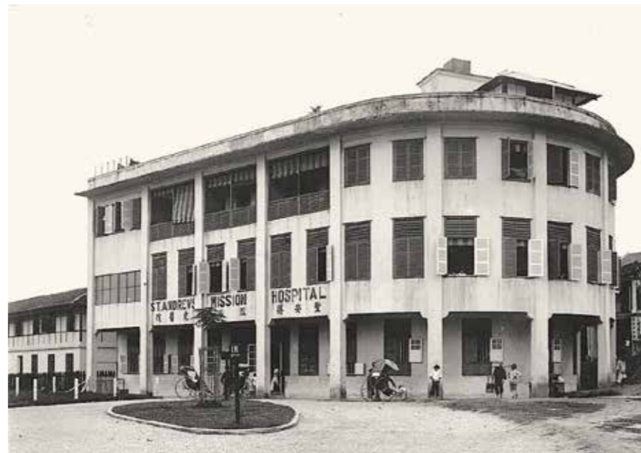
St Andrew's Mission Hospital at Erskine Hill, photographed in 1938. Designed in 1922 by Harry Robinson of Swan & Maclaren, the three-storey concrete frame building provided accommodation for 50 in-patients with additional quarters for the European and Asian staff on the top floor. The flat roof afforded recreational space for both staff and patients. Courtesy of St Andrew's Mission Hospital.
