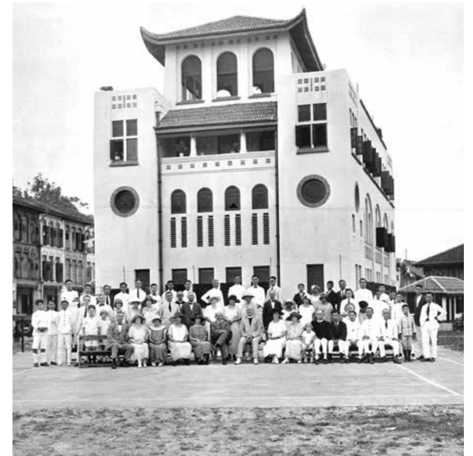
(Top) Denis Santry’s building plan of the proposed church and recreation rooms for the Telok Ayer Chinese Methodist Church, 1923. Building Control Division Collection, courtesy of National Archives of Singapore. (Above) Telok Ayer Chinese Methodist Church was consecrated by Bishop Titus Lowe on 25 April 1925. Designed by Denis Santry of Swan & Maclaren, it was a modern four-storey, concrete-frame building that was part-Byzantine and part-Chinese in design. Lee Brothers Studio Collection, courtesy of National Archives of Singapore.
