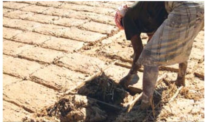
Putting mud mixture into the mould.
